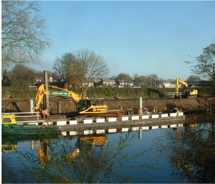
River bank repairs at Clifton – piles being set into river bank, and accumulations of silt being stripped off bank tops
