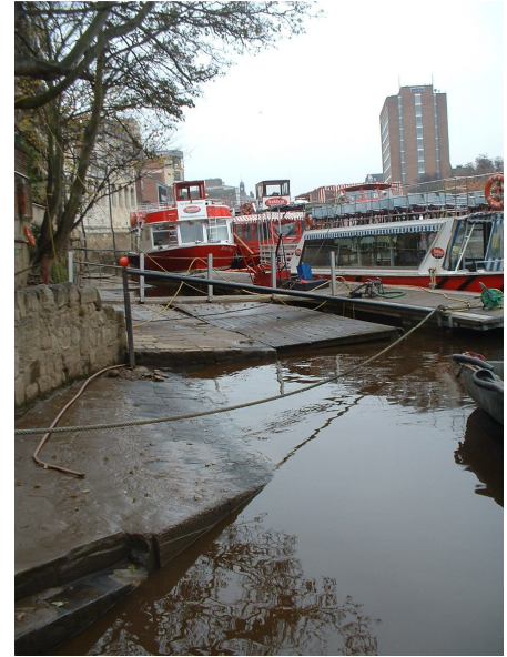
Lendal Boatyard where scouring by the river has created need for repairs
